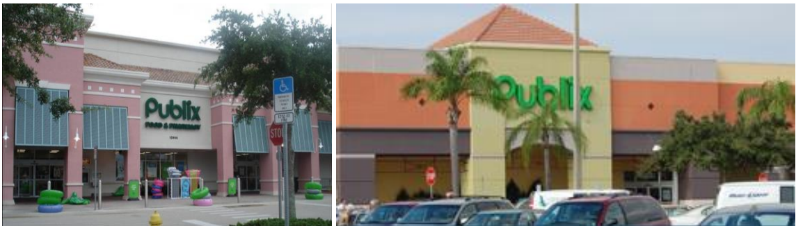
Figure 24: Bonita Grande Crossing and the Shoppes at Pelican Landing are both neighborhood centers anchored by Publix.
